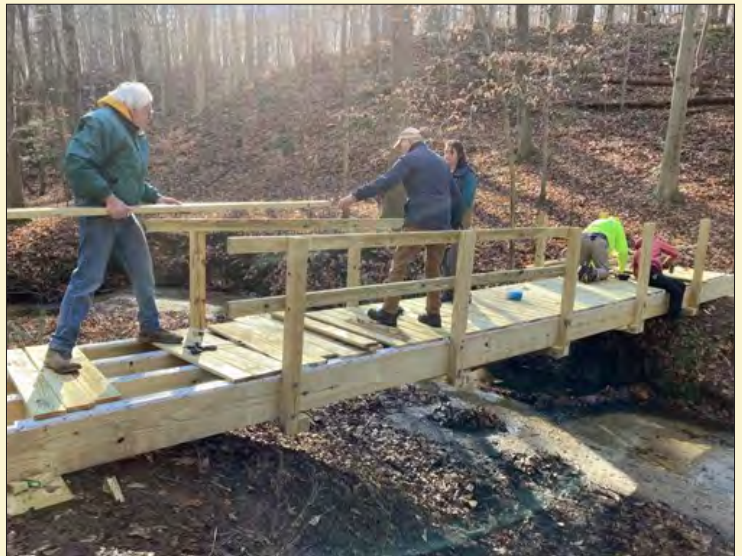
Above: Constructing the frame for the 16-foot bridge.
