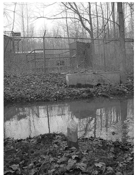
View Across Parkers Creek to Old Wastewater Treatment Plant
