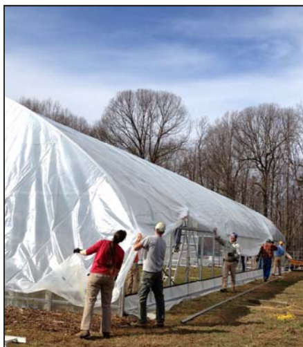
Pulling the cover on the High Tunnel. ACLT staff photo.
